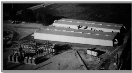
Energy Storage Peaker Substitution
